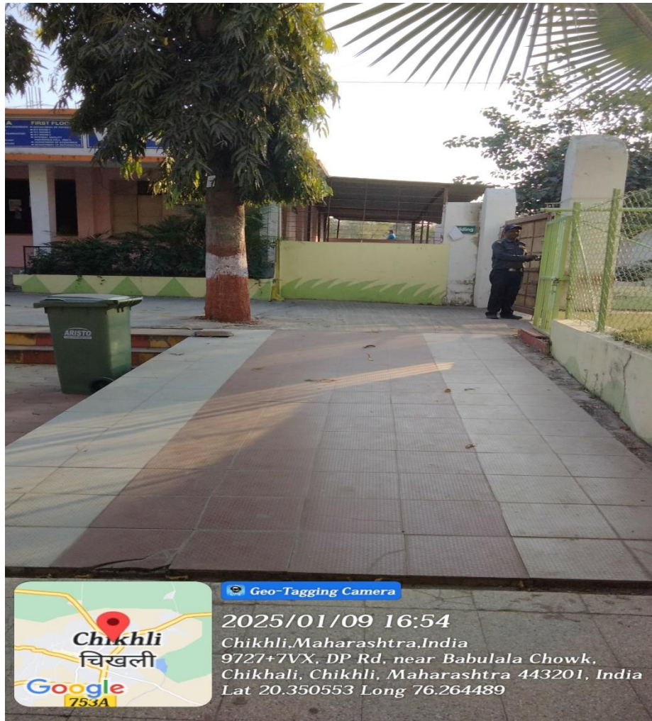
Divyangjan-friendly, barrier free environment: Ramp1 to office
