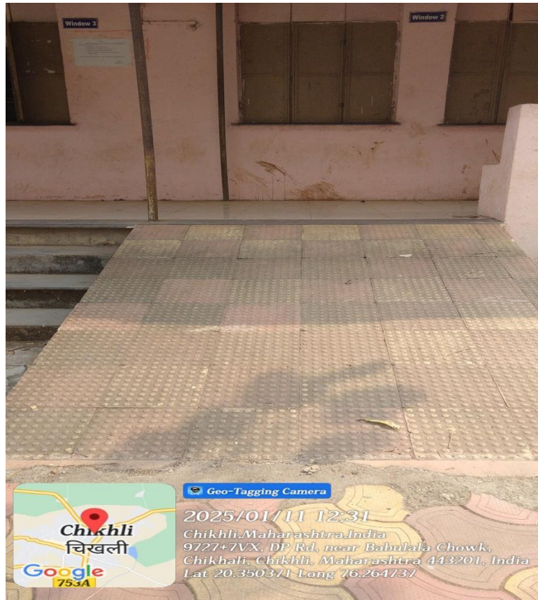
Divyangjan-friendly, barrier free environment: Ramp 3 to Administrative
